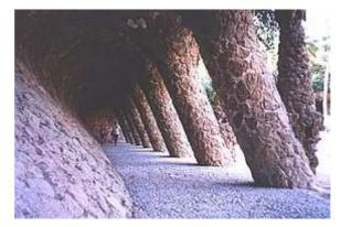
*Figure 53: The tilting of these columns is not solely an aesthetic decision, but follows the direction of the forces exerted by the load (Gaudí, Parc Guëll).*
